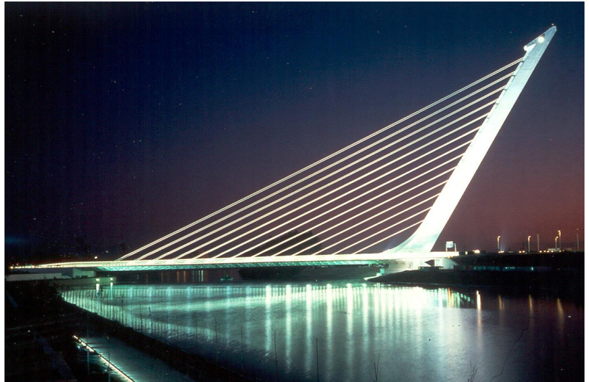
Alamillo Bridge, Seville, Calatrava
